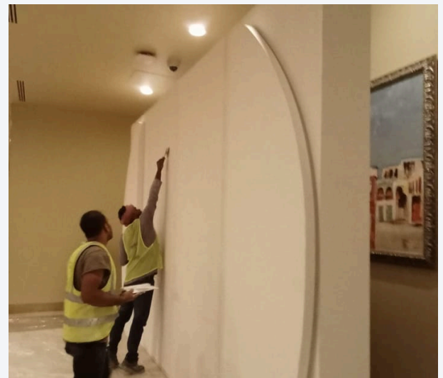
Fixing the curved wall panels.
