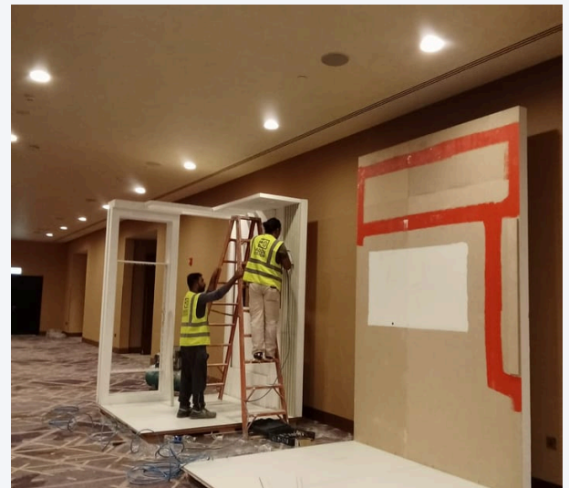
Setting out the walls in the ballroom.
